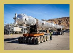
on the vessel during transport. The vessel was delivered to 600 ton and 350-ton hydraulic cranes for standing and final set to foundation. The transport, although short, was highly technical and involved extensive planning and was executed flawlessly.
