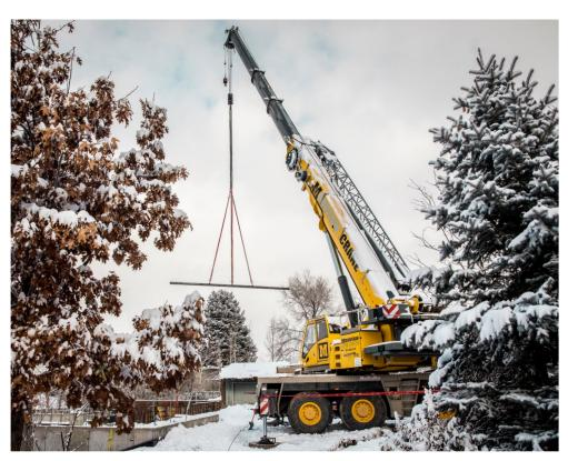
Fresh snowfall made for a scenic job-site in Salt Lake City recently. Using our Grove 115 ton, All Terrain crane, we placed an angle iron and 7 concrete beams approximately 16,000 lbs at this new construction, residential project.
