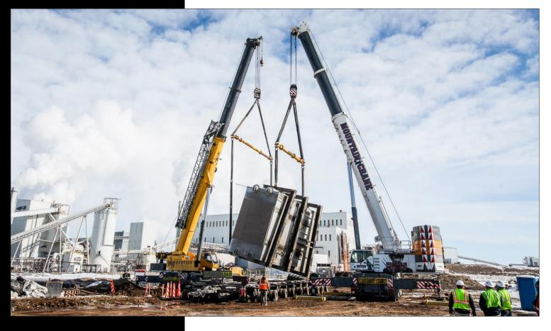
The engineering department at Mountain also provided a great deal of help to ensure we had appropriate ground bearing pressures, the proper rigging, and proper crane sizing to make for a successful job.
