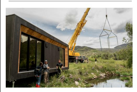
Talk about a quick turn around! This home was built completely in a factory, brought to the site, and our team did the heavy lifting. Our 200 ton crane and crew installed this modular home in no time at all, leaving the structure move-in ready! The home was built by Modal Living and is totally customizable for cabins, rentals, and recreation. Glad to be a part of this scenic job site!
