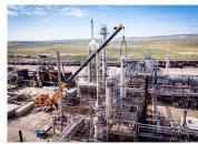
In August, Mountain Crane utilized the new Liebherr 1750t crane to place the new LEF tower in Sinclair, Wyoming.
