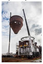
Mountain Crane Service performed a unique lift in January, using a Grove 550, a Liebherr 500, and a Grove 275. Working with RMF, Mountain Crane used the three cranes to place a large spray dryer filtration system.
