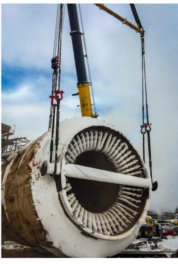
Mountain Crane recently had the opportunity to work with the Salt Lake City Tesoro Refinery to move a 280,000 pound boiler. In addition to providing the engineering on the lifting lugs system for this project, Mountain Crane was pleased to provide the lift plans for the crane. While looking at this project, we chose the 2250 CR and the 6300L AT as the right tools for the job.
