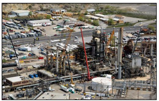
Mountain Crane Service recently completed a major turnaround project at the Tesoro Refinery located in North Salt Lake. These shutdowns require extensive amounts of engineering lift plans, project management, and crane work. Planning for this project started last summer.
