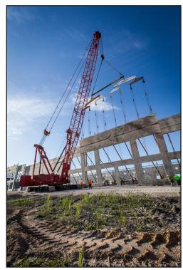
wide panels required 32 pick points, seven spreader bars, and 24 snatch blocks to pick and set into place. The Manitowoc 2250 required more boom than usually required on a tilt up in order to facilitate the additional required headroom because of the multiple levels of rigging.
