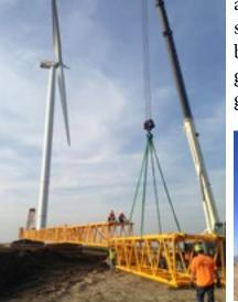
and then the hub/rotor assembly was installed. This was projected to take 10 days, but was completed in 3 days thanks to a great assembly team, operators and riggers.
