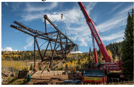
This A frame metal structure once stood as the head shaft tressil at the Daly West Mine in Park City, Utah. The tressil is 85 feet tall and weighs 76,000 pounds. The mine shaft was 2100 feet deep.
