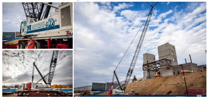
Mountain Crane is thrilled at the opportunity to help with the construction of the new Maverik Stadium at Utah State University in Logan, Utah. Mountain Crane is currently providing the crane for the erection of the steel for the press box structure using our Linkbelt 278 300t lattice truck crane.
