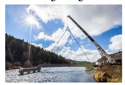
Mountain Crane and Cannon Builders recently worked together to upgrade a bridge in beautiful Ashton, Idaho. The 112 foot long girders were set by a Grove GMK 7550, weighing in at about 88,000 lbs. each. A 100 ton dolly was also used for transportation of the old bridge.
