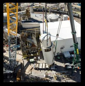
Mountain recently performed a turnaround project that involved our LR1600 cralwer and LTM1750 all terrain cranes. The highlight of the event was removing a cold reheat exchanger and replacing it with a new one. We even got our SMPT Goldhofer trailer in the mix!
